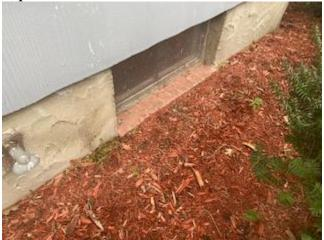
It is recommended window well(s) be installed at any basement/crawlspace windows where the soil is less than 6 to 8 inches below the window.
