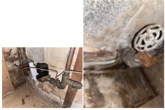
**Interior Supply Pipes:** The visible portions of the piping for the branch lines are copper but the main to the street is galvanized metal. If there are galvanized pipes, these tend to build up material on the interior as they age, reducing flow rate and rotting from the inside. It is recommended you budget to replace these pipes in the near future.
