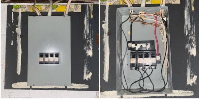
**Conductors:** The branch wiring is copper BX and copper romex, as viewed from random outlets and switches and the panel box(es).
