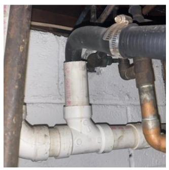
If there are galvanized pipes, these tend to build up material on the interior as they age, reducing flow rate and rotting from the inside. It is recommended you budget to replace these pipes in the near future.
