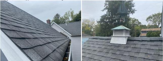
The roof covering is in acceptable condition with no leaks detected. The roof has a remaining life expectancy of up to approximately ten years.
