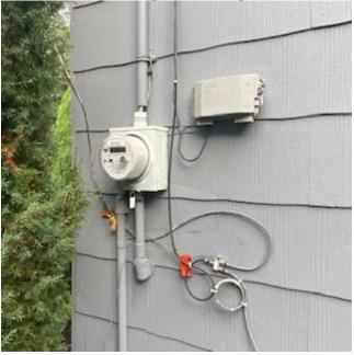
Service line: The electric service line entering the house is a type 3 wire capable of supplying both 110 and 220 volts. It is in acceptable condition.
