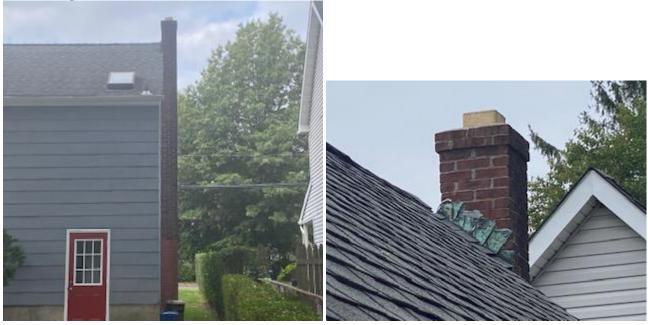
As the full length cannot be inspected, you may wish to have it further evaluated by a licensed chimney contractor. It is recommended caps be present on chimney flues to help prevent possible water and animal entry.
